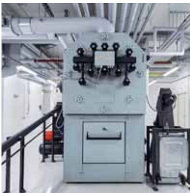
Vitoflex 300-UF pellet boiler with a heating output range from 300 to 950 kW
