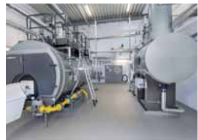
Vitomax HS steam boiler (left) with TWA-V total thermal deaeration system (right)
