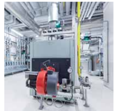
The Vitocrossal 300 gas condensing boiler (type CR3B) is designed for an output of up to 787 kW and serves as a peak load boiler.
