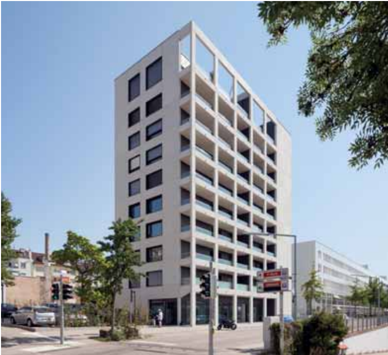
This fully modernised high-rise apartment building in Pforzheim relies one hundred percent on renewable energy sources.
