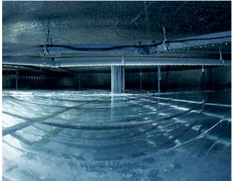
The crystallisation processes in the ice store can be visualised via camera transmission.
