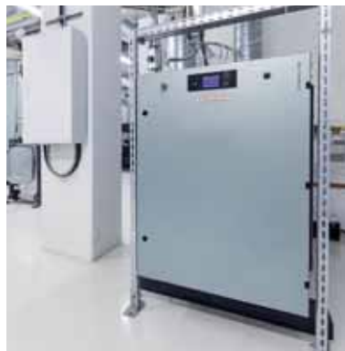
Vitobloc 200 EM-20/39 CHP unit with outputs of 20 kW el and 39 kW th
