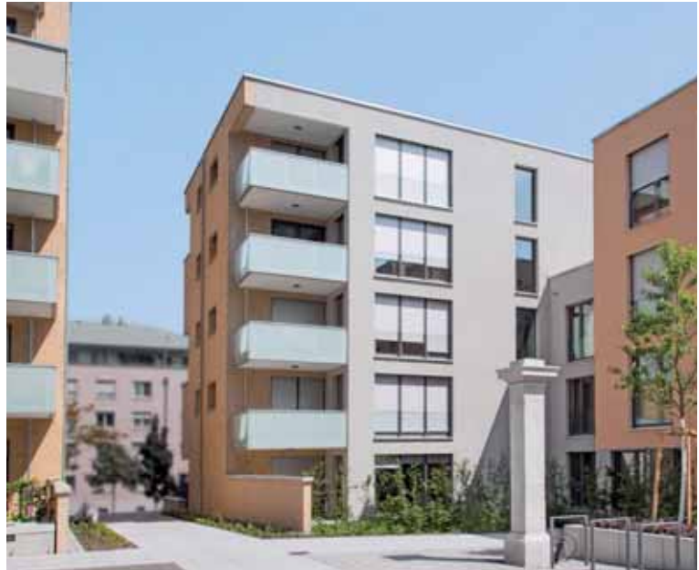
The Rosenstein Quarter in Stuttgart: 500 apartments have been constructed here according to the principle of sector coupling.
