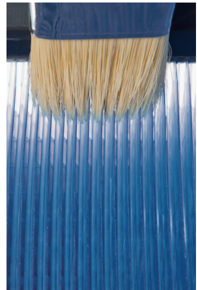
Straightforward servicing of the mechanical ventilation system (in this case the Vitovent 300-W): Visual inspection of the filters (top left) and filter replacement in the case of severe contamination. The heat exchanger can be cleaned with a brush, vacuum cleaner or jet spray.
